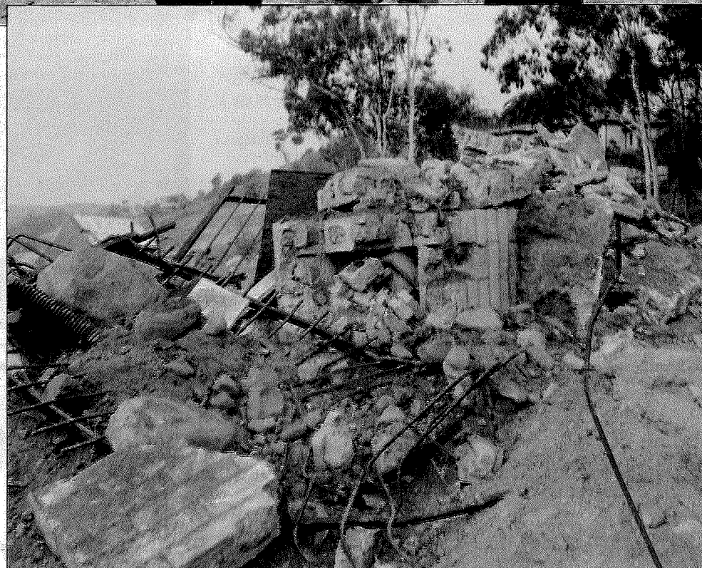
(Top) RSF's Gene Magre was not able to save his home during the 2007 fires, which has prompted his new interest in a business to help prevent home loss to fires. William Leon, Gene Magre and Clay Merritt stand on the corner of Magre's lot. (Bottom) All the remaining debris of Gene Magre's house; the property overlooks a Rancho Santa Fe valley. The house was lost in the October fires in 2007 along with other nearby homes. Photos/JonClark
