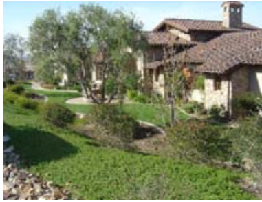
A home within our district demonstrating proper vegetation management and fire-resistive construction
